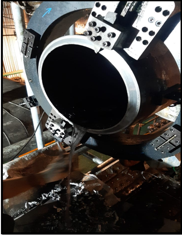
Cold Cutting & Bevelling
